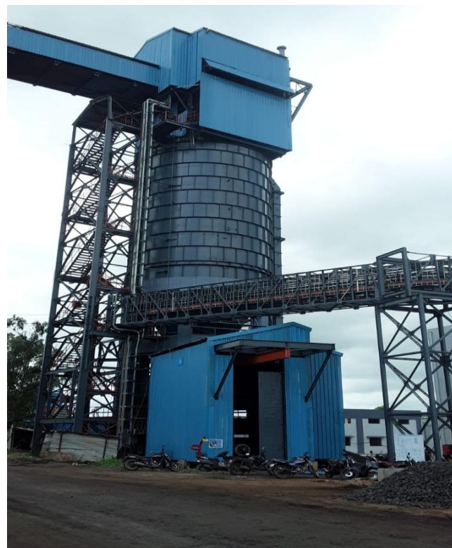
Cladding at Surge Hopper at Bhatadi
