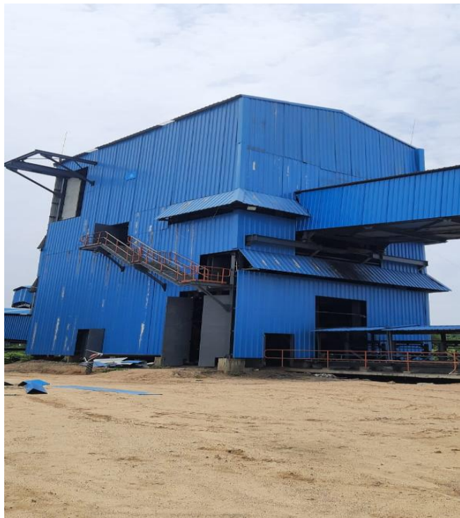
Cladding at Junction house – JH01
