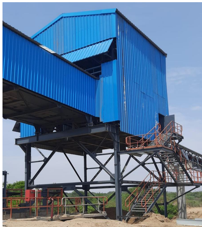
Cladding at DST-02
